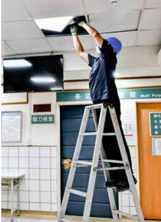
Members of the Dalin Tzu Chi Hospital Engineering Department replace traditional fluorescent tubes with energy-saving LED tubes.
