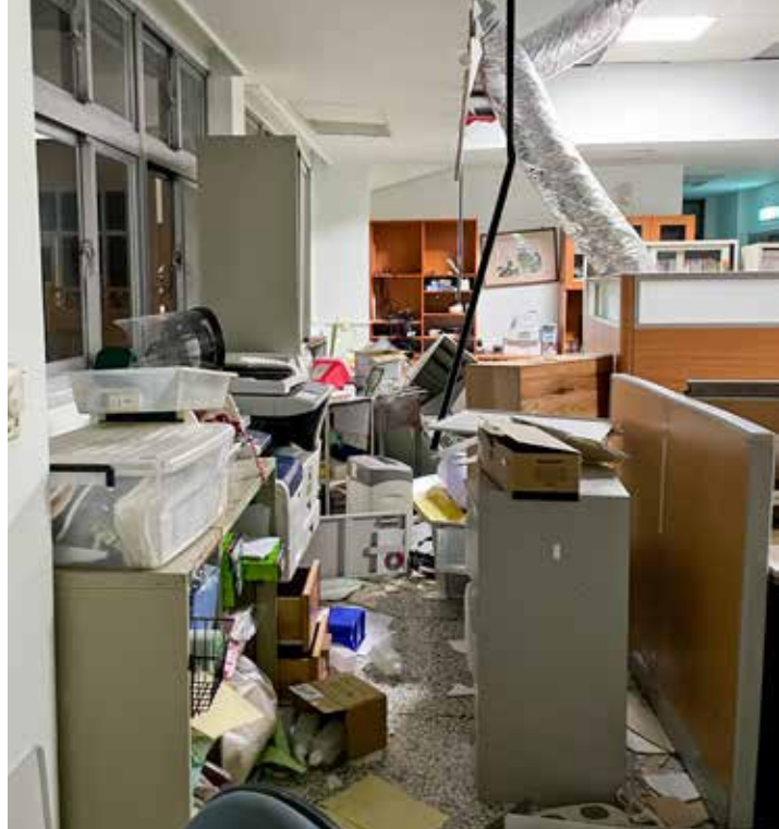
Chaotic office area on the 7th floor after the earthquake.
