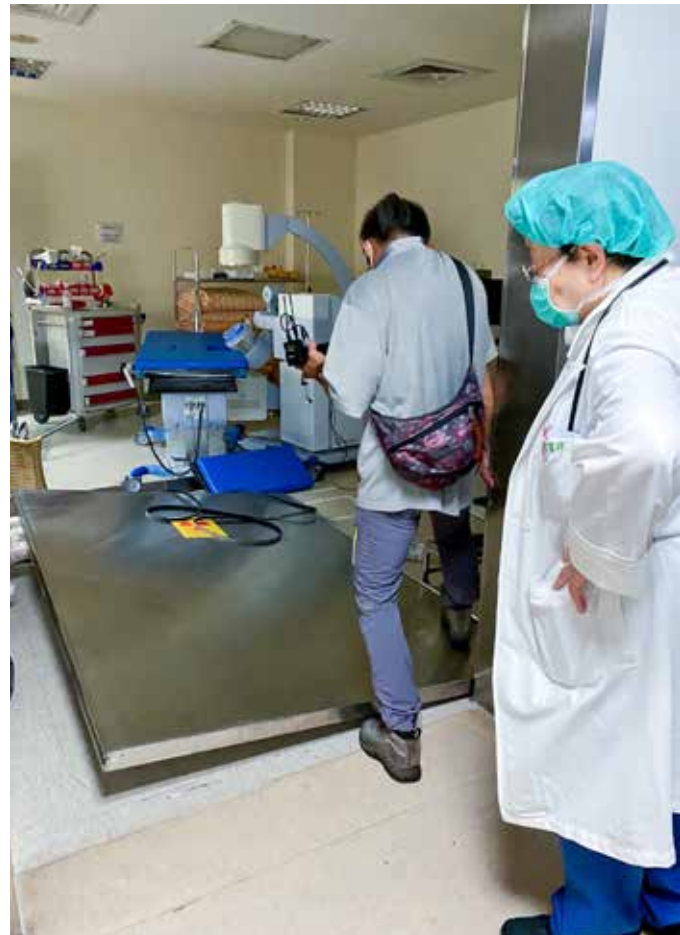
The over 100kg-heavy lead door of the shockwave room of Yuli Tzu Chi Hospital has been knocked down by the powerful earthquake. Fortunately, there are no casualties. Superintendent Chen Yen-Pi on the right.
